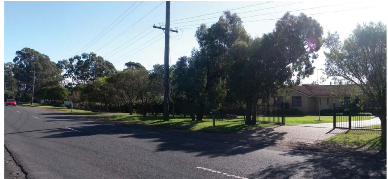
Fig. 2.2: Low density residential development along Smalls Road
